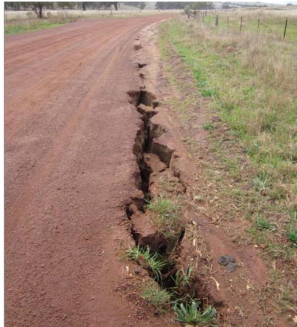
Fig. 4.10 Isolated Surface Cracking parallel to longwall tailgate above Longwall 26 at Ulan Coal Mine, 410m void width, 1.38m maximum observed subsidence, 240m cover (Ulan Longwall 26 End of Panel Subsidence Report)
