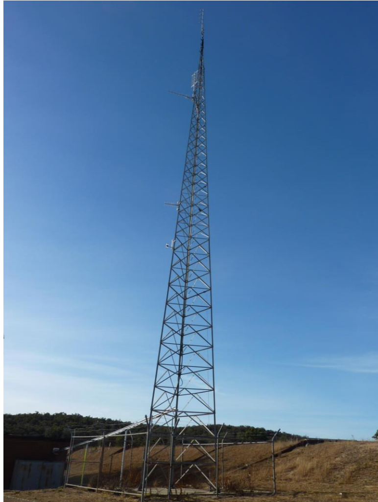
Figure 4 telecommunications tower and dam embankment
