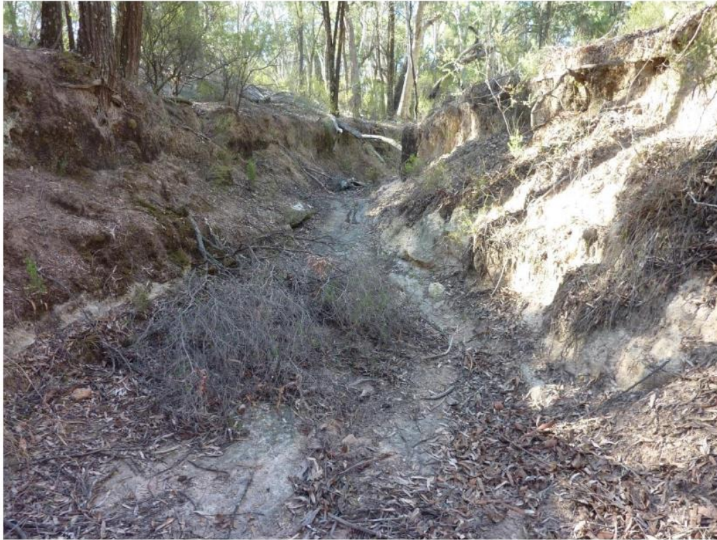
Figure 2.3 - Photographs showing Drainage Line 2 (Source: MSEC, 2021)
