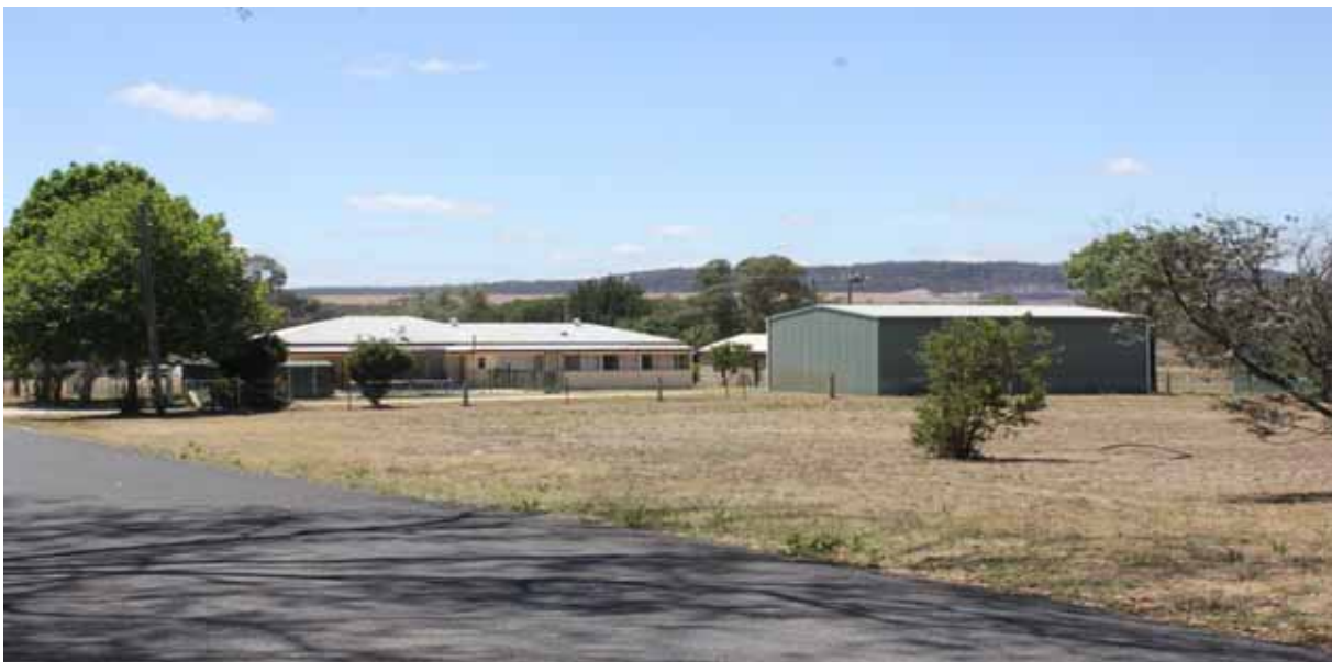
Figure 4.9 Views to Open Cut 1 from VP4 currently obscured by rehabilitated overburden emplacement area
